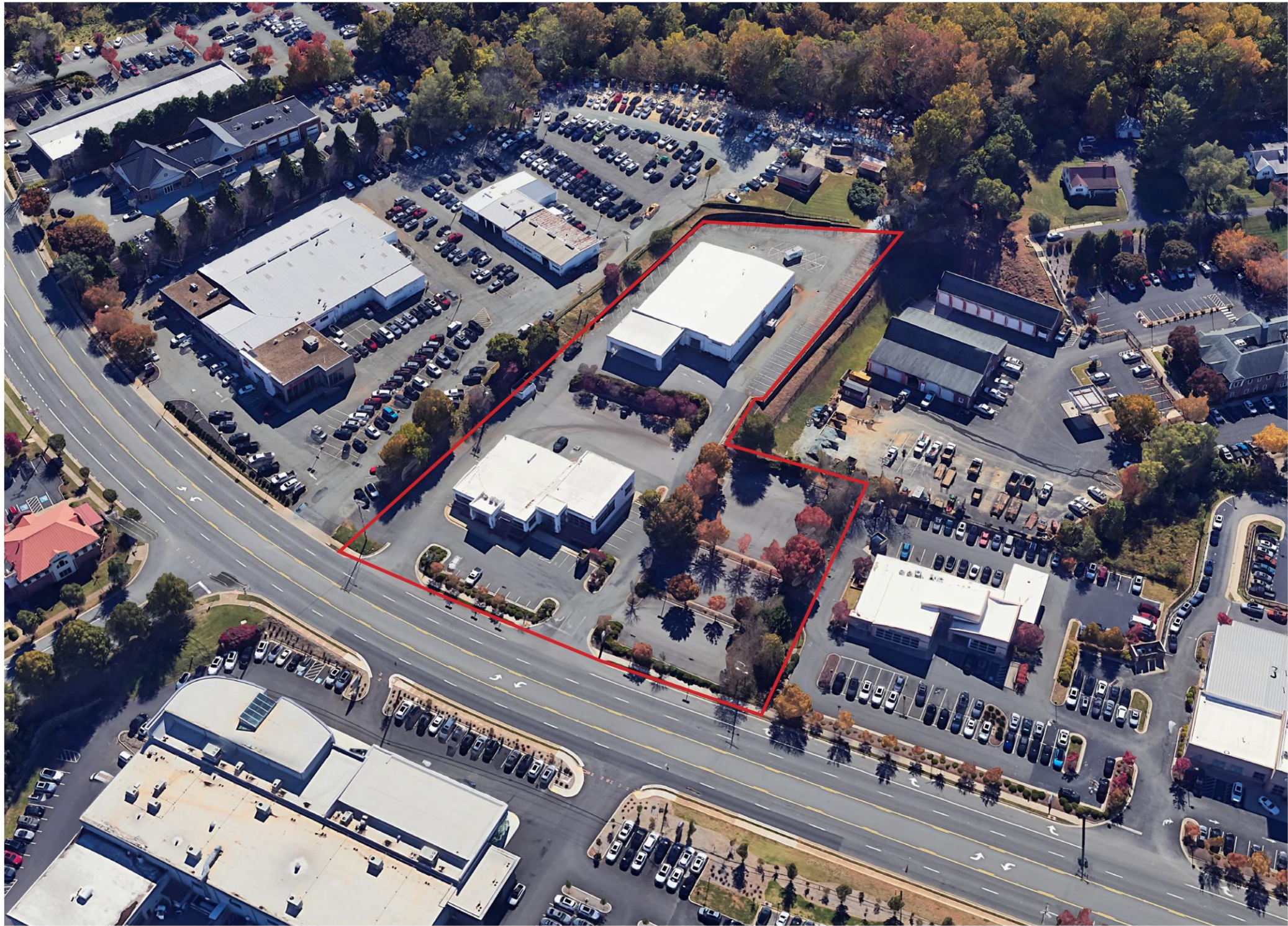
View from Richmond Rd 250
